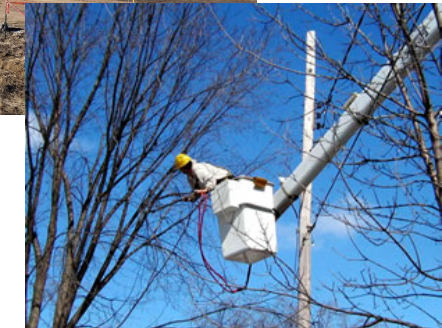
Tree trimming underway
